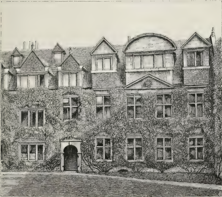
Fig. 13. West end of North side of Sir Robert Hitcham's building.
